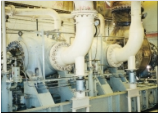
T100-C on Solar Centaur Gas Turbine Engine.
